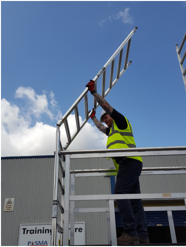
11. Fit an additional set of frames as shown and secure interlock clips.
