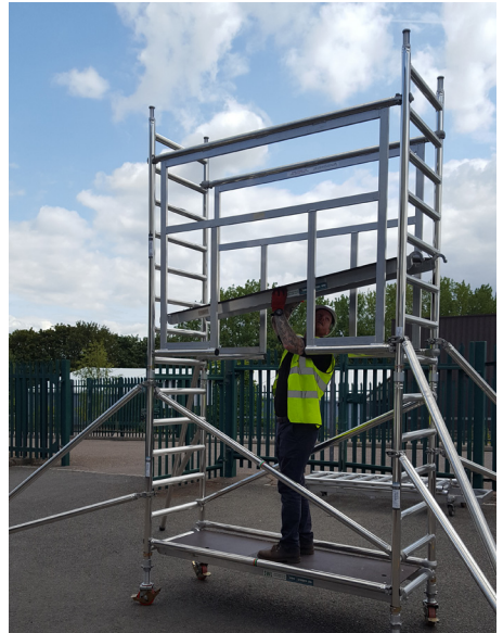
10. Position the trapdoor platform to the rung, 6 rungs down from the top of the frame.
