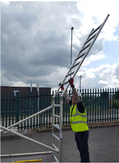
7. Add a set of frames as shown and engage the interlock clips.
