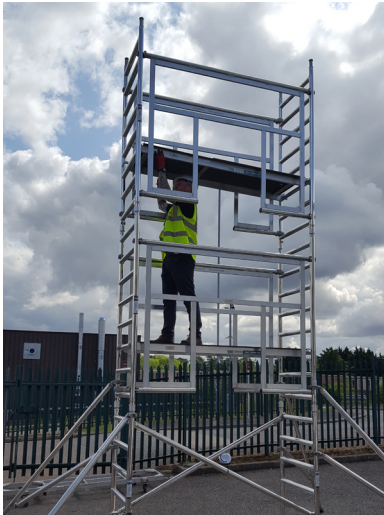
13. Position the trapdoor platform to the rung, 6 rungs down from the top of the frame.
