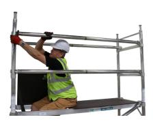
From a seated position remove 4 x guardrails making sure you never stand on an unprotected platform.
