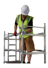
Unclip 4 x Horizontal braces from the far end of the trapdoor platform.
