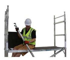
From a seated position descend down the tower to the next platform or ground. Ensure you always have collective protection around you when standing on any platform.
