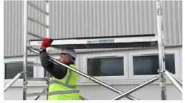
11. From the temporary platform, fit 1 diagonal brace to 3rd rung down and fit trapdoor platform over the hook. Offset platform to oneside and run the diagonal brace away from the trapdoor.
