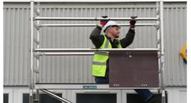
13. From a seated position using the through the trapdoor (3T) method. Fit 4 horizontal braces, hooks facing outwards to the frame upright.
