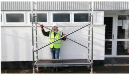
8. Fit 2 more diagonal braces to continue in a regular pattern on the 3rd rung leaving room for your horizontal braces to fit on the upright.
