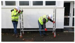
4. Fit 2 horizontal braces to the verticle member of the frames above first rung. Horizontal braces fit on from the inside of the tower facing outwards
