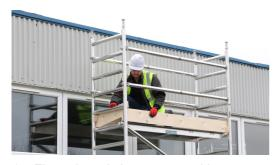
17. Fit toe-boards in correct position
