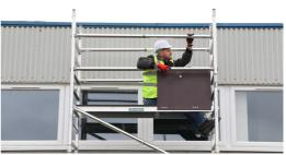
16. From a seated position, using the 3T method, fit 4 horizontal braces above the appropriate rungs to the frame verticles, hooks facing out.
