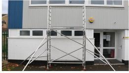
12. Remove temporary platform and the 4 horizontal braces. Relocate the 2 diagonal braces from 3rd to 1st rung.
