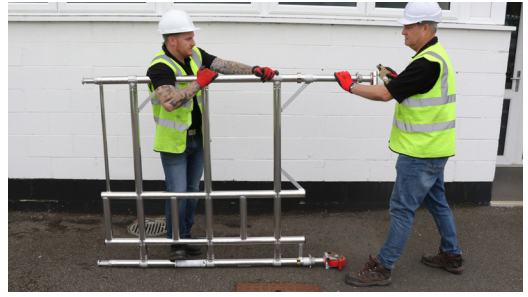
2. Insert 2 adjustable legs and castor wheels into each base frame
