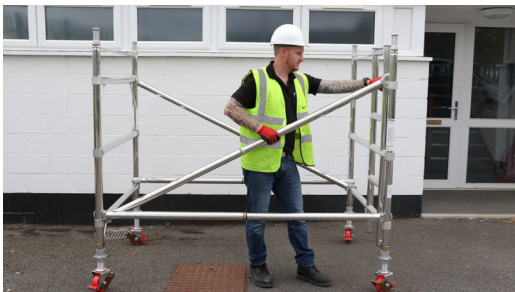
5. Fit 2 diagonal braces from the 1st rung to the 3rd rung in an alternate pattern.
