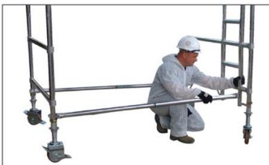
2 Fit in 2 horizontal braces to the vertical member of the frames, as low as possible, below the 1st rung. All horizontal braces fit on from inside the tower facing out.
