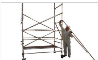
11 Secure stabilisers as soon as possible to increase tower stability. Check tower kit list to ensure the correct stabilizers are fitted.
