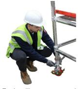
For levelling purposes only, the buttress legs can be adjusted by turning the leg nut as shown.
