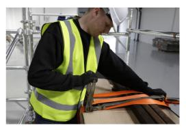
8. Secure the ballast to the platform(s) to avoid accidental removal.
