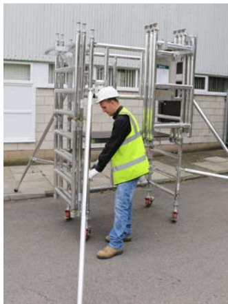
19. Fit 4 stabilizers, one on each upright of the tower.
