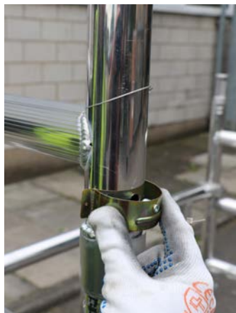
13. Engage interlock clips.
